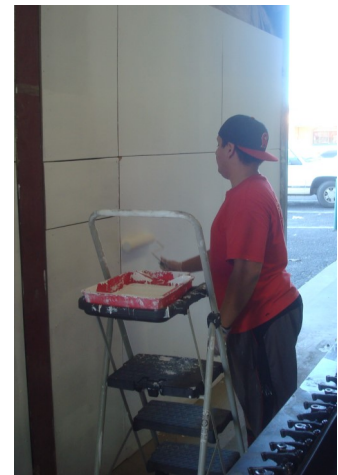
Youth trainee, Nicholas Barraza , painting wall panels installed by Dennis Gibbs
