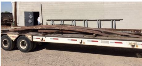
Rail being loaded for transport to the new 36 th St. preservation yard.
