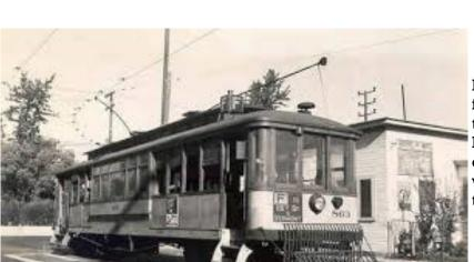
Here is the same design car in a later configuration operating in Los Angeles. Note the ends have been enclosed. These were large cars of 44.5 ft. in length and had a capacity of 54 passengers seated. LARY was narrow gauge with 42 inches between the rails.
